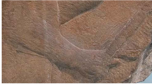
FIGURE 8. Detail showing the use of a point chisel to rough out the surface of the stone
