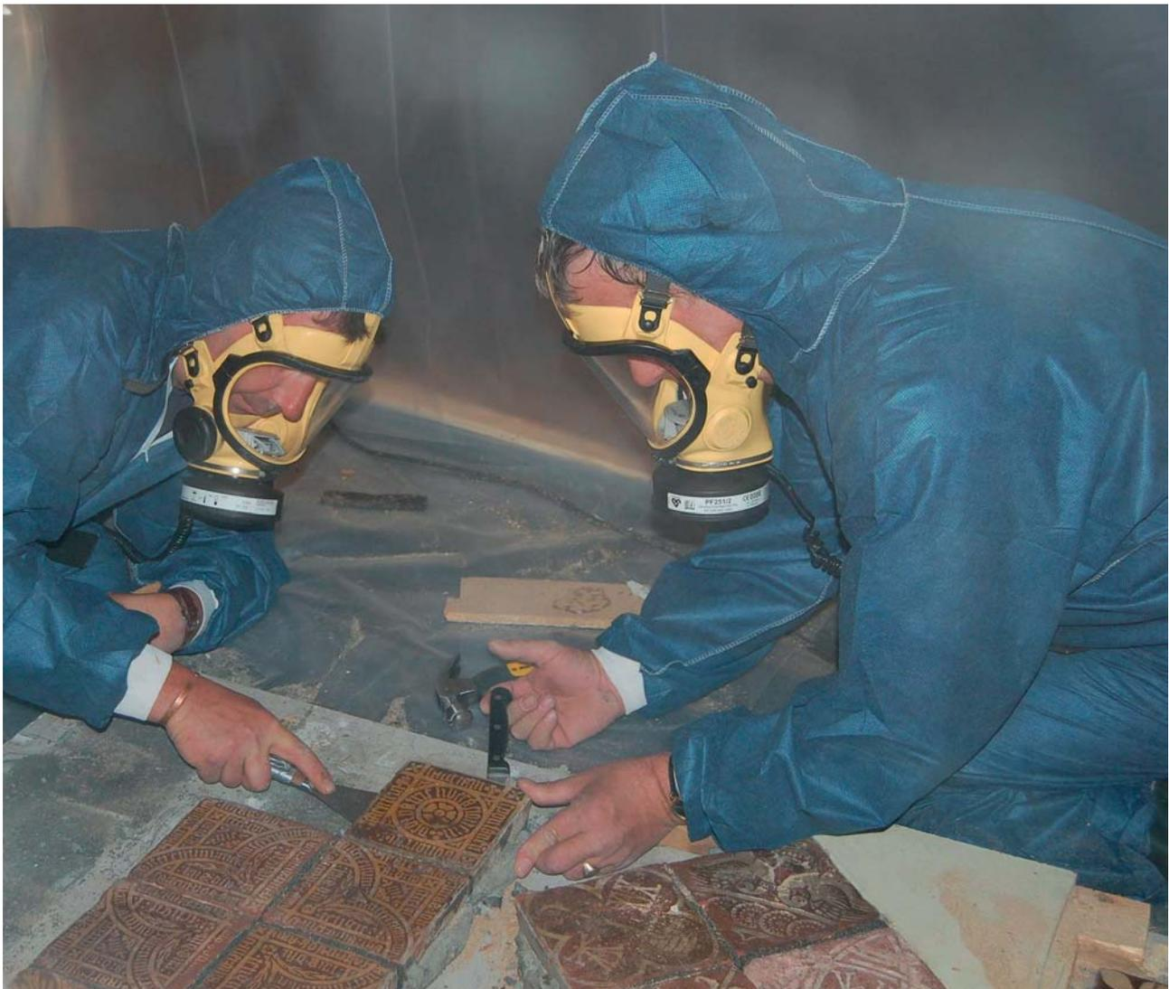
FIGURE 6. Specialist asbestos contractors, wearing protective clothing and working in the isolation tent, gently prising the Malvern tiles and the dark grey rubber adhesive backing off the Asbestolux board
