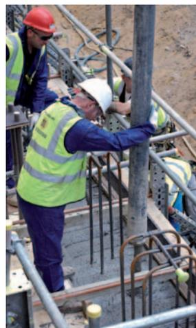
Pouring concrete to form capping beam
