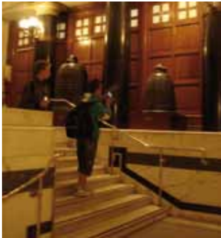
The lowest flight of the North stairs
