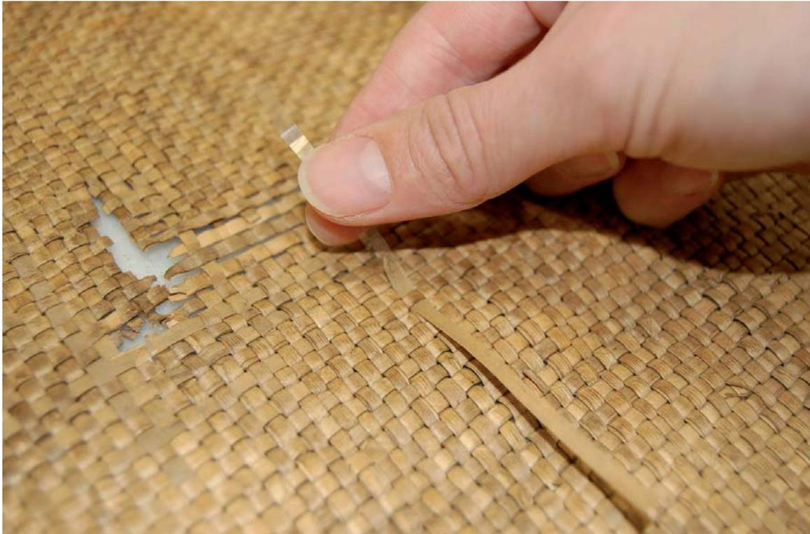
FIGURE 9. Using a 'needle' cut from heavyweight Melinex<sup>®</sup>, a mulberry paper support strip is woven across a weak area. To the left of the damaged area, already incorporated repair strips are visible
