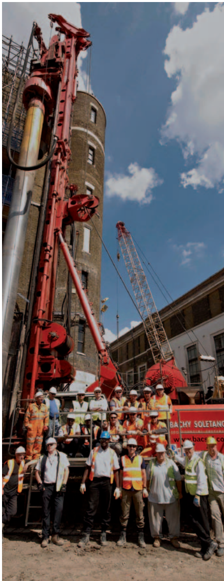
The Bachy team before leaving the site in August
