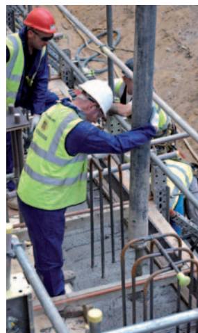
Pouring concrete to form capping beam
