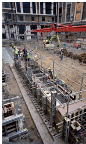
Installation of capping beam
