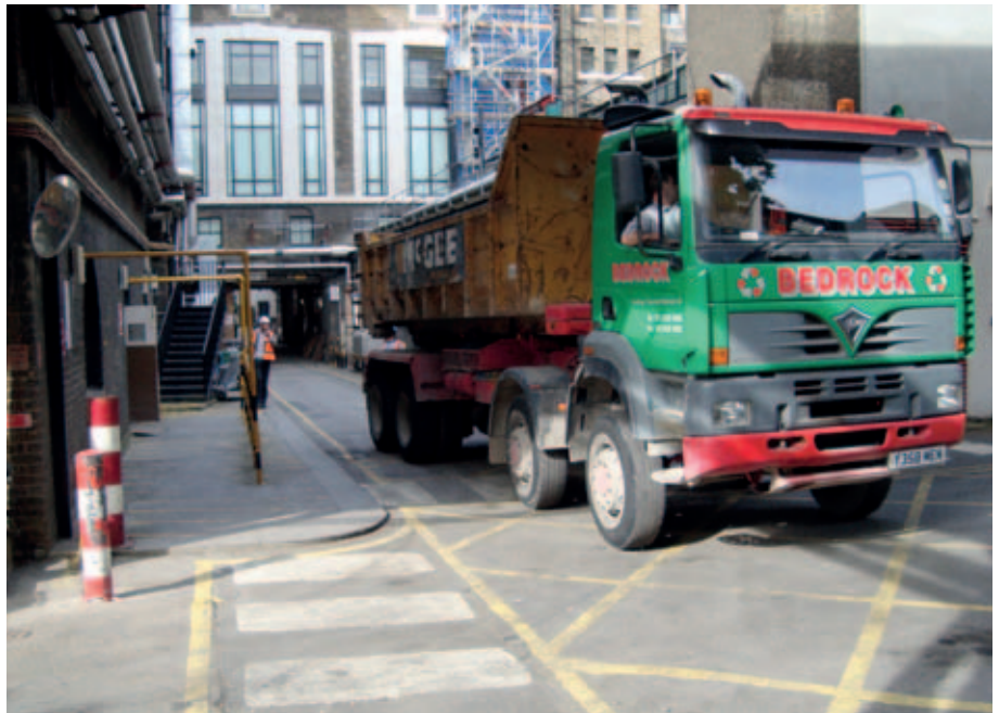
Demolition truck leaving site
