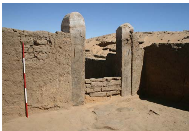
Entrance porch to villa, with sandstone doorjambs, and later brick blocking, still in situ
